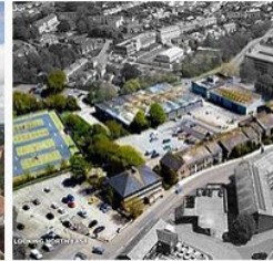
Cornwall Council Pydar Street Development
